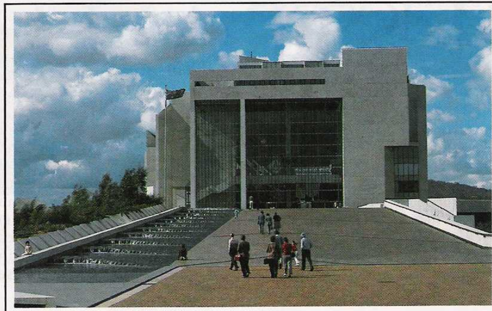
The High Court typifies the modern design of Canberra's newest buildings. The entry ramp is used for important ceremonies. (Photo by Robert C. Taylor)
