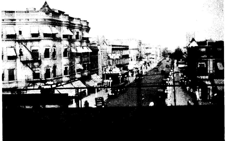
Wilson Avenue, Chicago, in 1917, looking east toward the lake, from Sheridan Road Elevated platform. The Armstrongs' first home after marriage was 1 1/2 blocks down this street.
