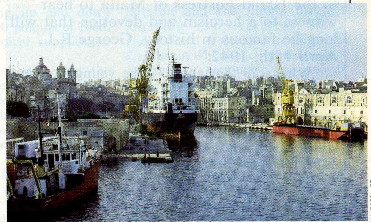
Malta's harbors and shipyards—still an important source of income.
