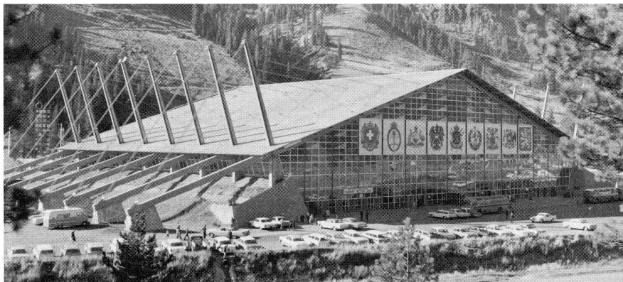
BELOW—Large fir trees and rugged mountain slopes enclose the place where God has placed His name.
