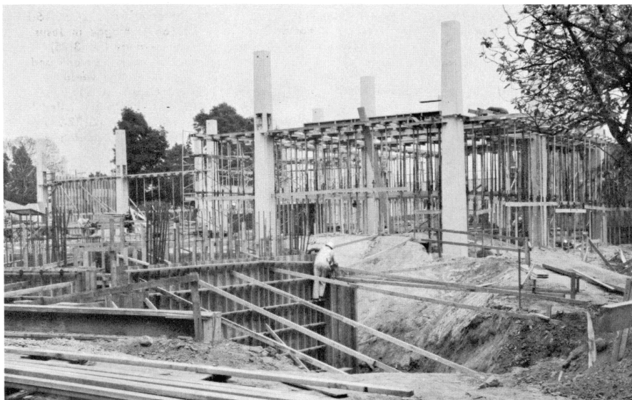
GOING UP —The pre-stressed concrete columns shown above will support an equal number of lightweight "umbrellas" of similar construction, which will become a part of the roof. The columns rest on foundational pillars extending 53 feet below ground level. Heavy-duty cranes will soon hoist the large roof beams—78 feet long—similar to those used in the gymnasium.
