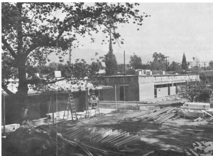
NEW SCHOOL —Rheem Manufacturing Company has construction well advanced for new grade school building. Made of modular components primarily for speed, cost approximates stucco-plaster.
